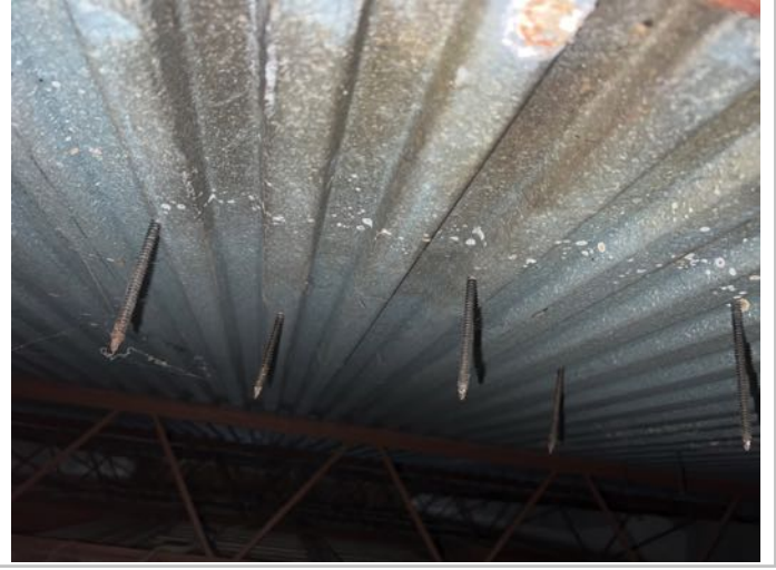
corrugated concrete deck form
